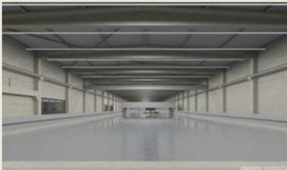
The new maritime research centre will also include a 30 m long, 30 m wide and 1.5 m deep wave basin in order to test off-shore and shore protection structures and wave and tidal energy converters under different environmental conditions. Having both the [towing tank](#) and wave basin within the same facilities will create an important synergy of talent and experience.
